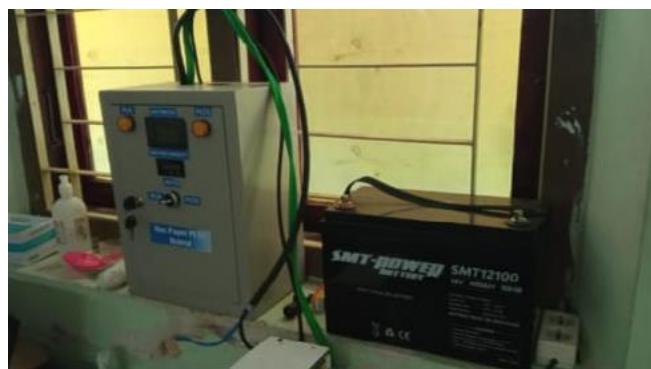
Fig. 3. There is only 1 unit of electronic device and battery as a PLTS charging source
