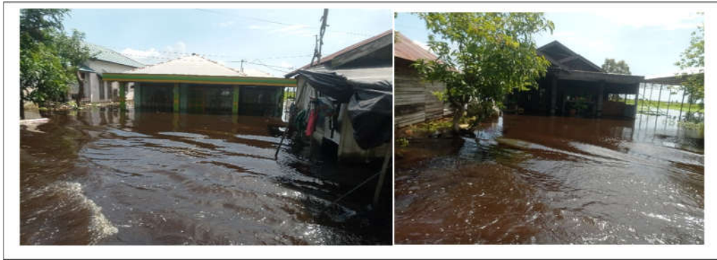
Fig. 1. House Submerged in Flood
