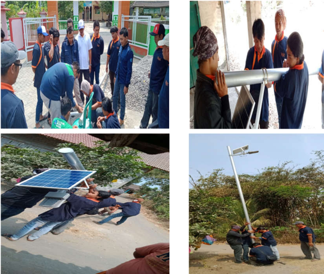
Figure 3. Practice of installation of PJU lights with solar cells
