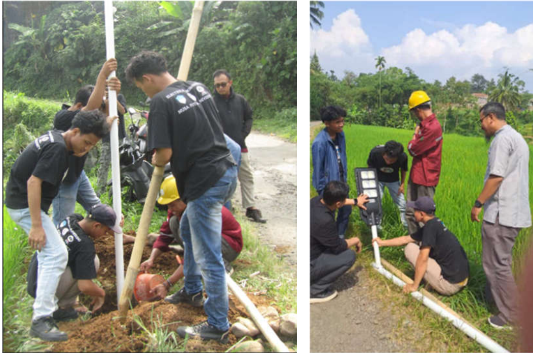
Fig. 1. Installation of solar panels
