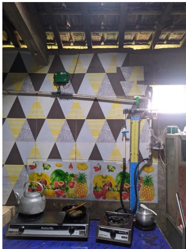
Fig. 4. Installation of a biodigester monitoring device
