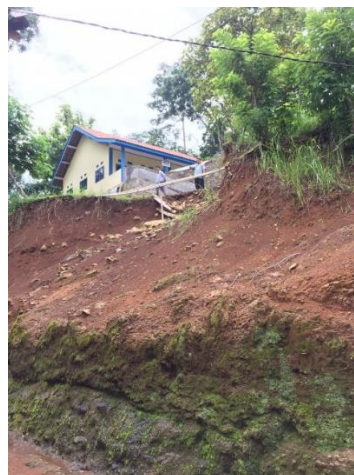
Fig. 1. Initial Location Survey
