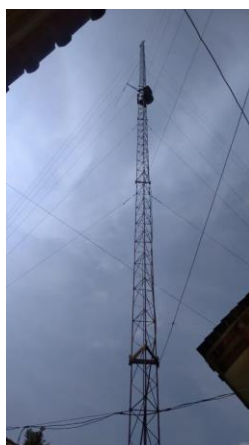
Fig. 5. Installing an outdoor FM radio antenna on the tower
